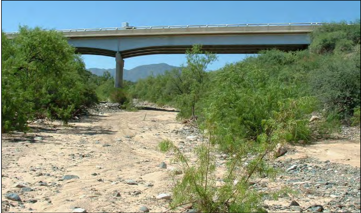
Figure 11: A large bridge spans Black Canyon on Highway 260 in Strand B (waypoint 008).
