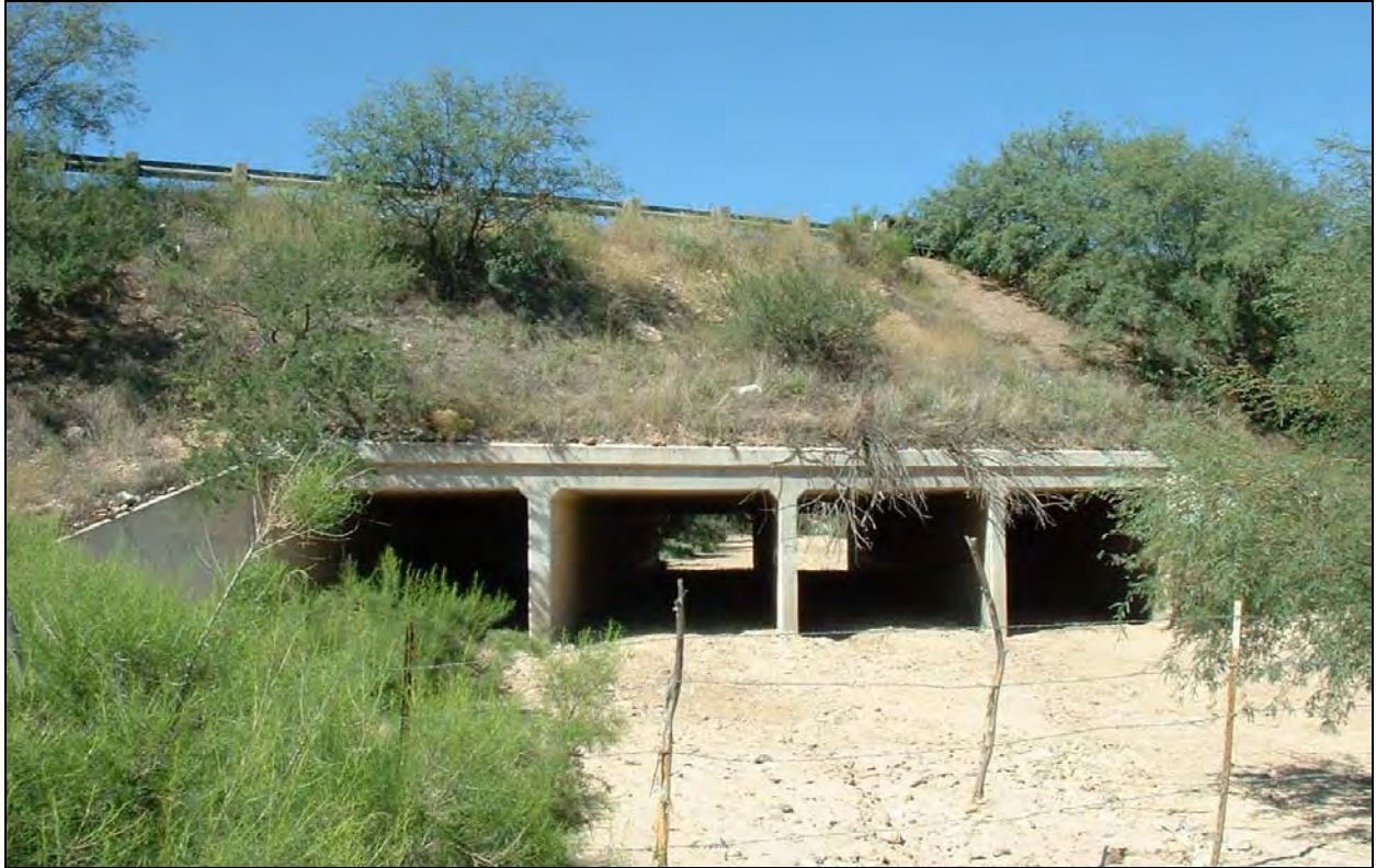
Figure 15: A 4-span culvert crosses under Highway 260 ½ mile south of Strand C (waypoint 003).
