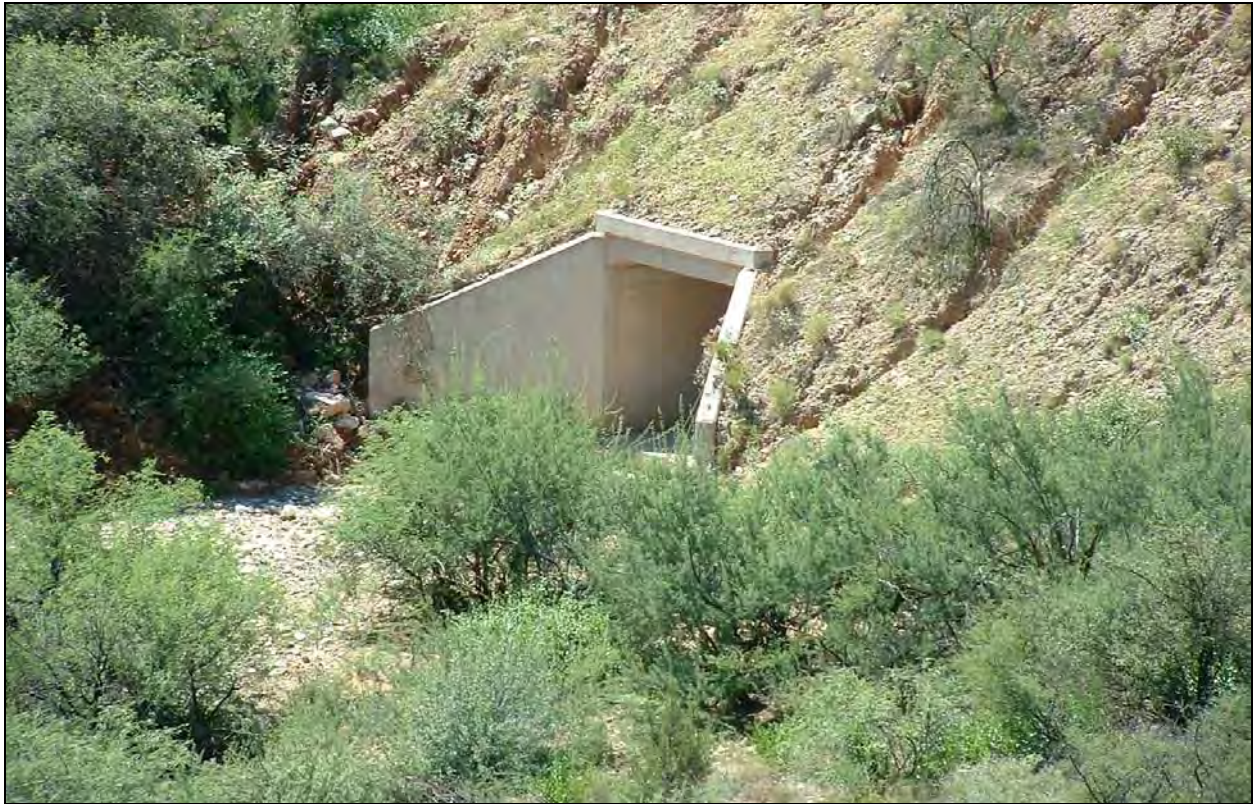
Figure 12: A small box culvert crosses under Highway 260 in Strand B (waypoint 009).
