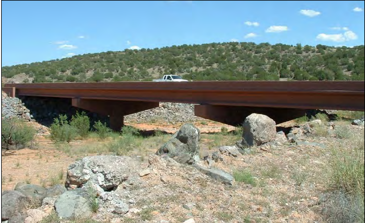
Figure 13: A large new bridge crosses along Hwy 89 over Spring Creek in Strand B (waypoint 010).
