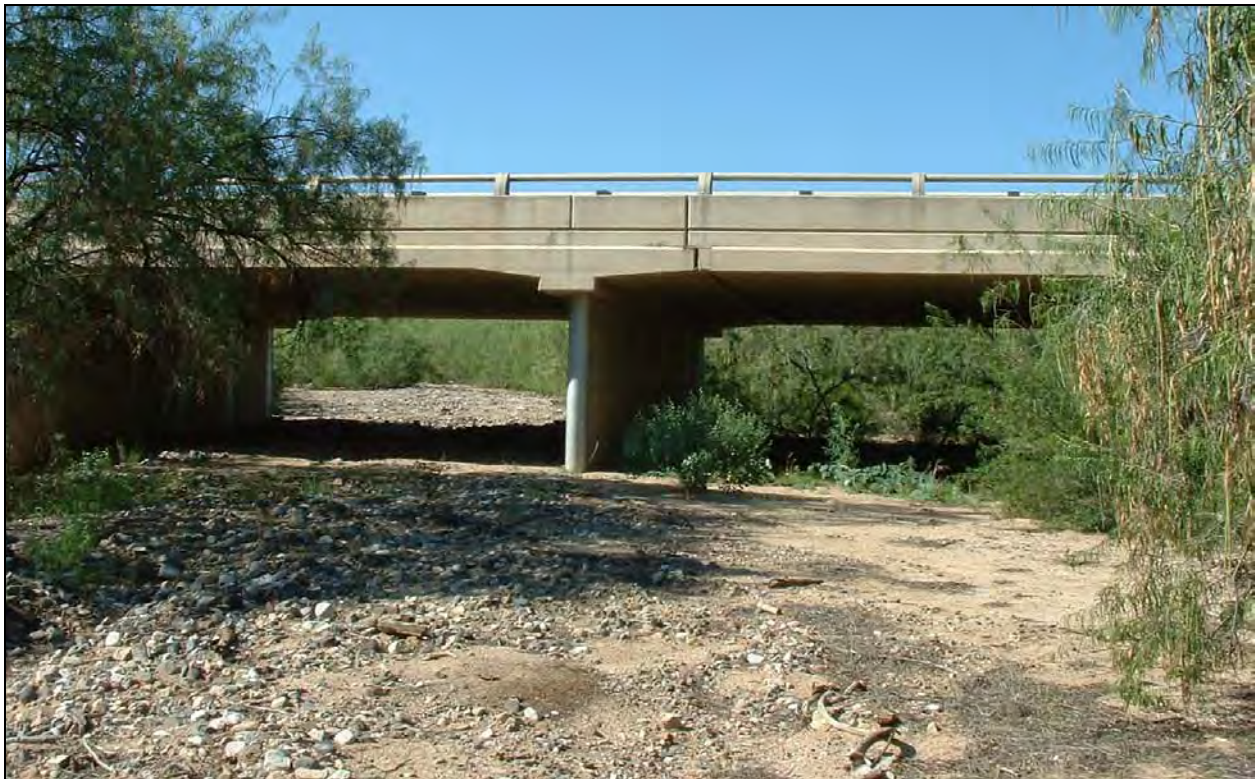
Figure 16: A large multispan bridge crosses over Cherry Creek on Highway 260 (waypoint 011).
