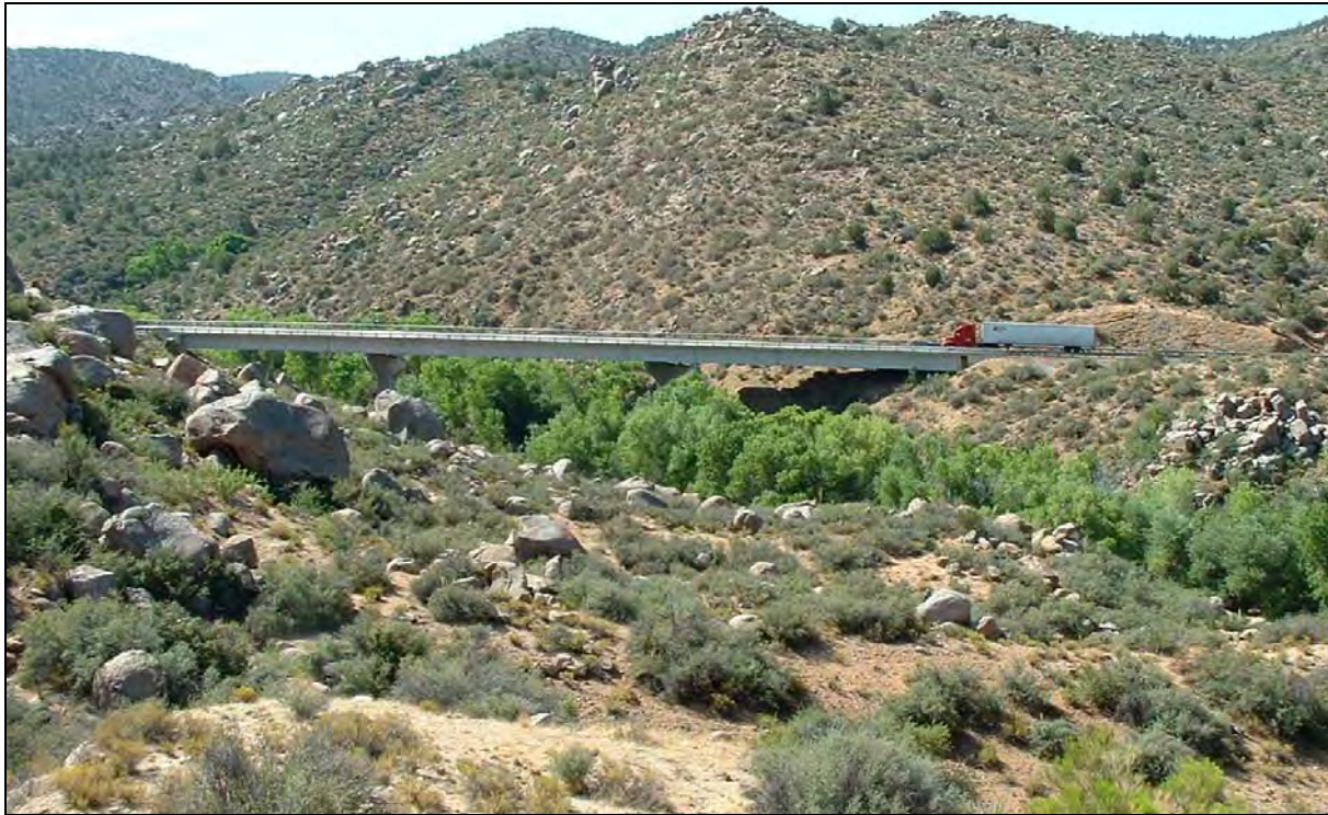
Figure 16: Large bridges in the eastbound lanes of I-40 cross Willow Creek in 6 locations between milepoints 83.1-86. This photo taken from waypoint 086 shows bridge at MP 83.75.
