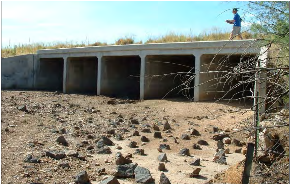
Figure 17: Looking southeast from waypoint 084, five 8x8 box culverts cross over Lookout Wash.
