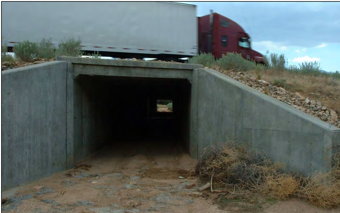
Figure 13: Looking southwest from waypoint 095, a single 10x8' box culvert runs under I-40. A dirt road runs through the culvert.
