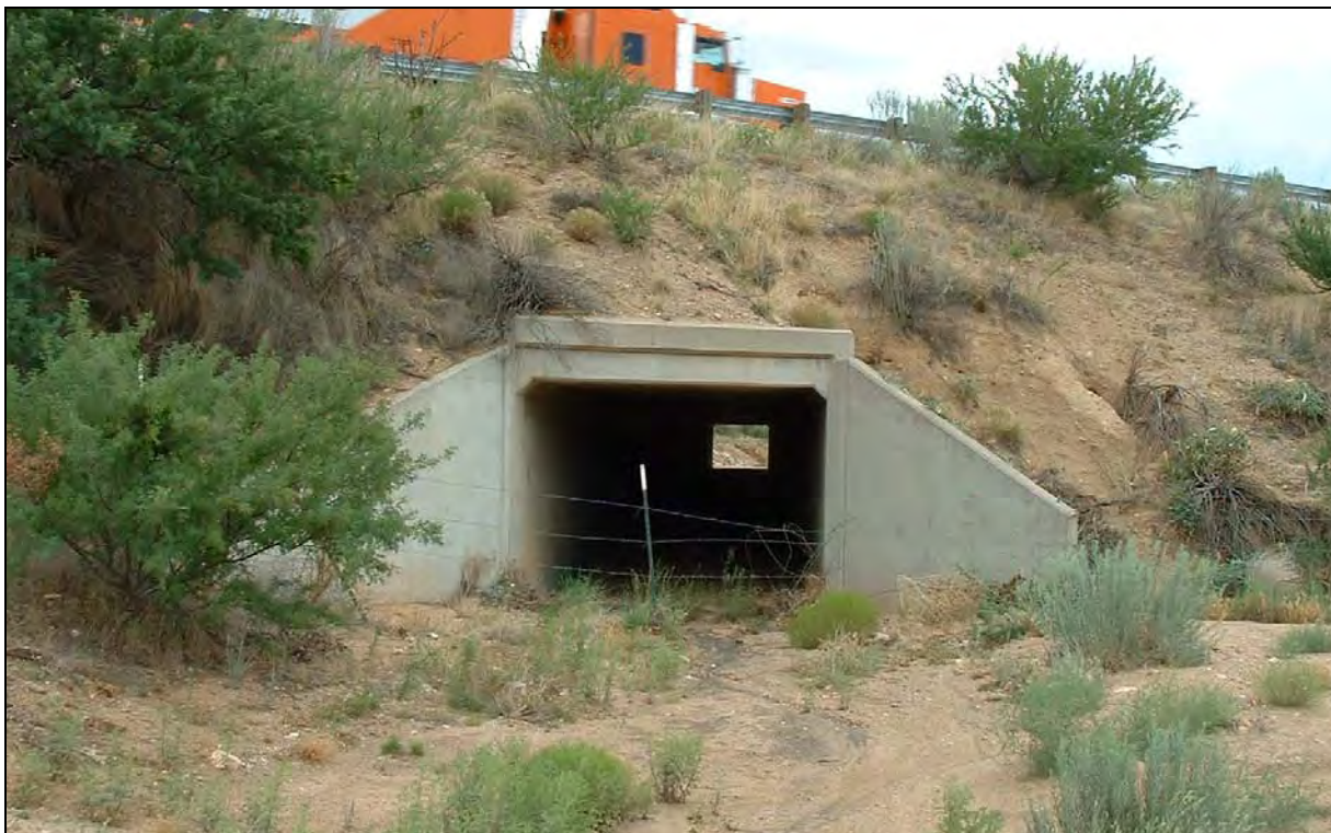
Figure 15: Looking northeast from waypoint 097, a single 8x8 ft culvert crosses under I-40.
