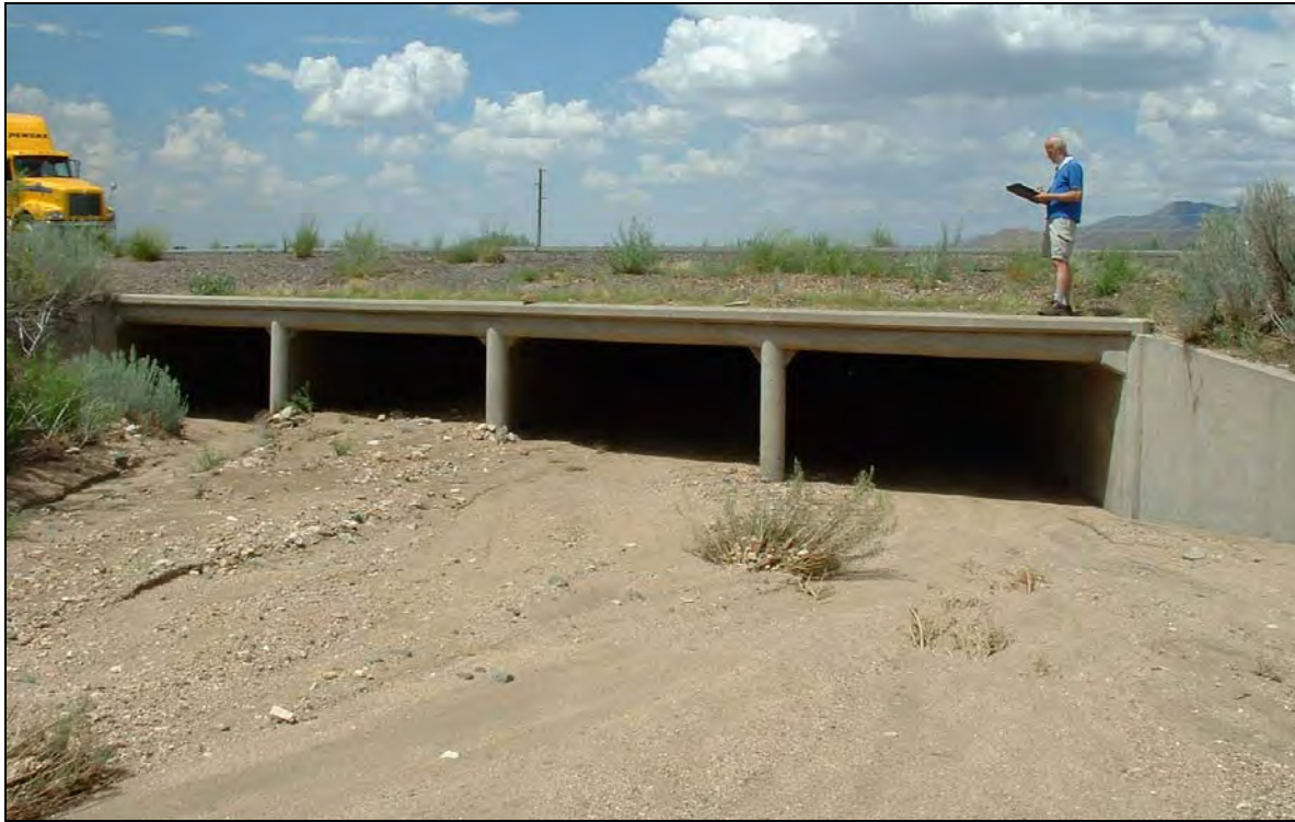
Figure 12: Looking north, four 4x10 ft box culverts provides only limited connectivity due to a heavily silted-in bottom (waypoint 094).
