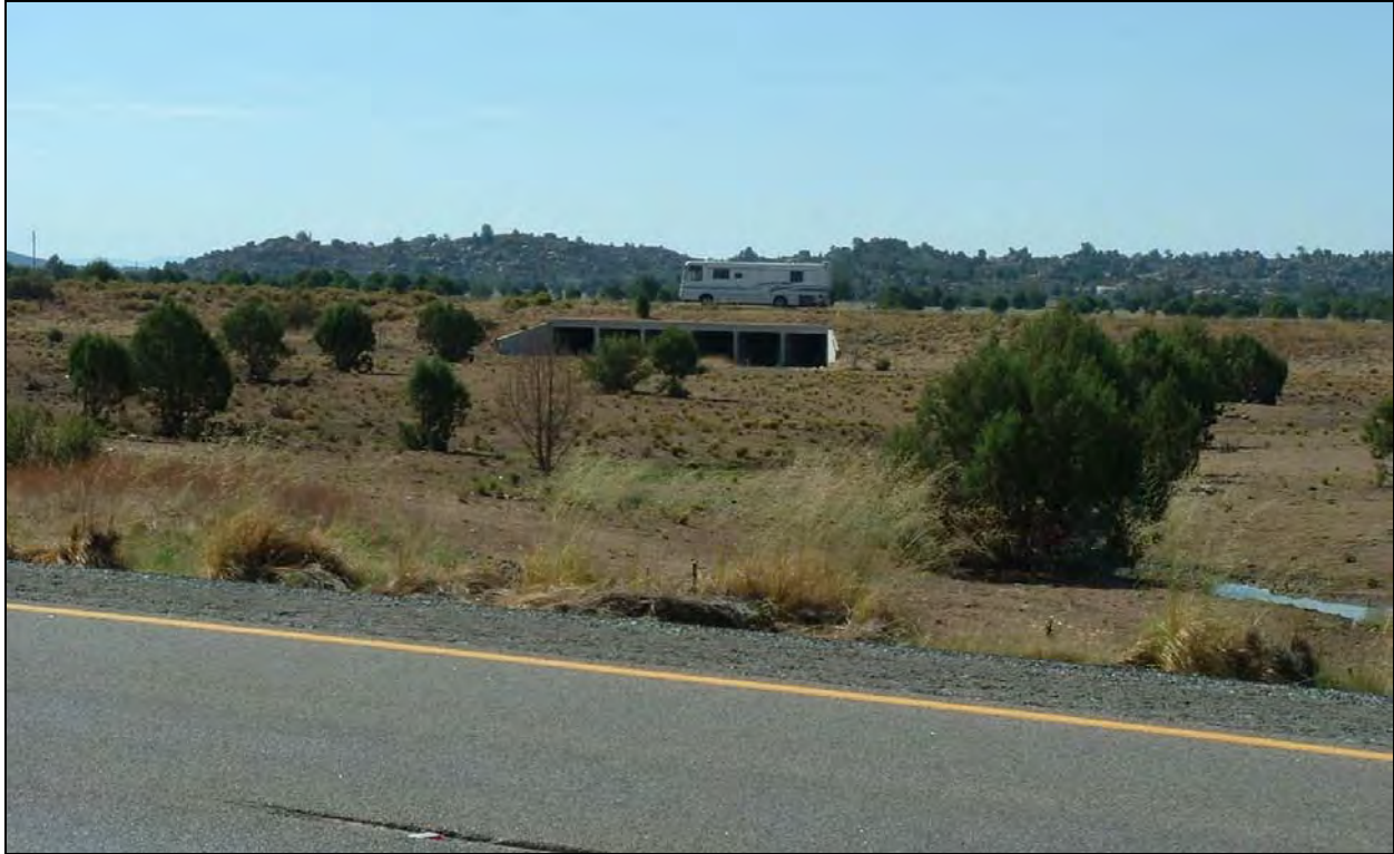
Figure 18: Six culverts cross under the westbound lanes of I-40 for the wash (bottom).
