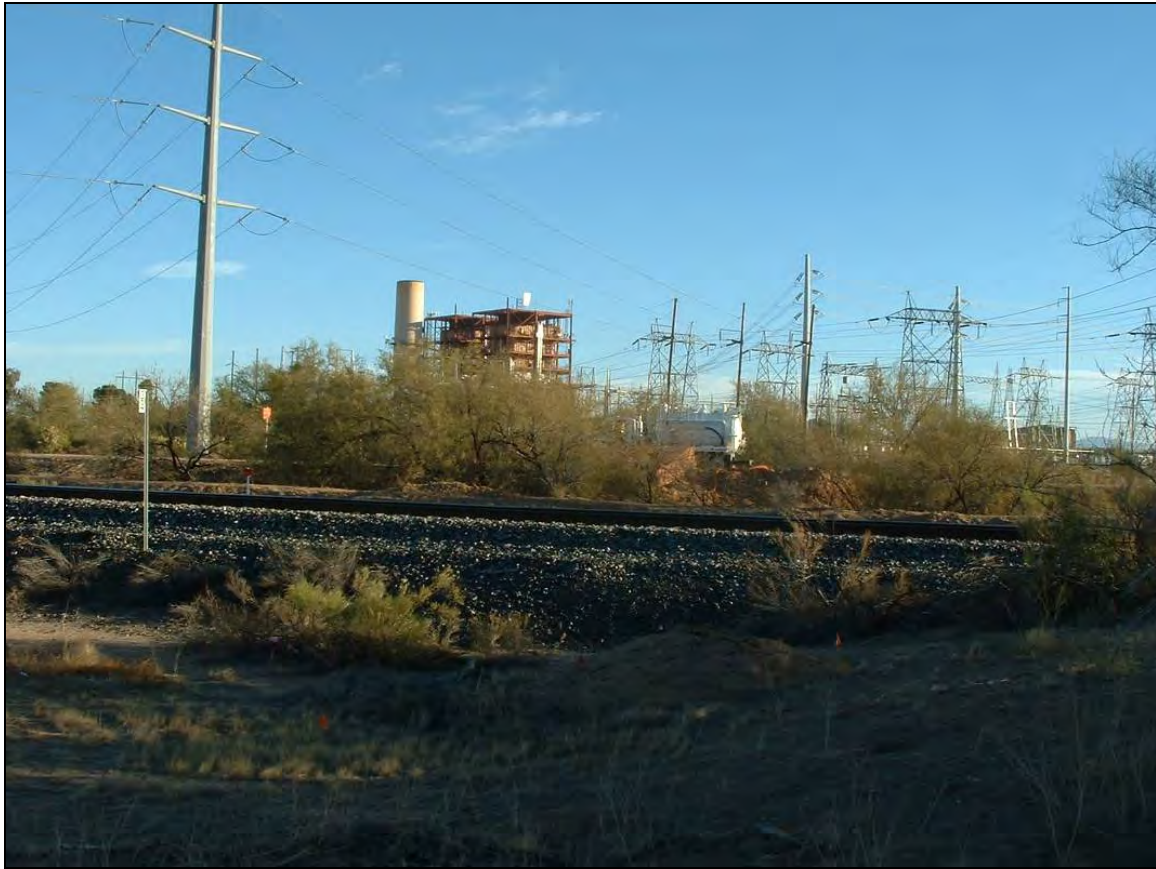
Figure 21: The Saguaro Power Plant borders the southern end of the Ironwood - Picacho linkage adjacent to I-10 (waypoint 72; azimuth: 38).
