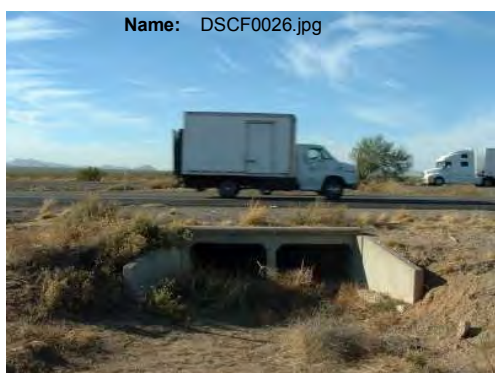
Azimuth: 220 Zoom: 1x Notes: Twin box culvert, each approx. 4x5 ft.
