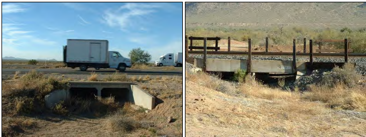
Figure 14: A small twin-span cement culvert (azimuth: 220) and a wooden railroad crossing (azimuth: 22) occur at waypoint 91.
