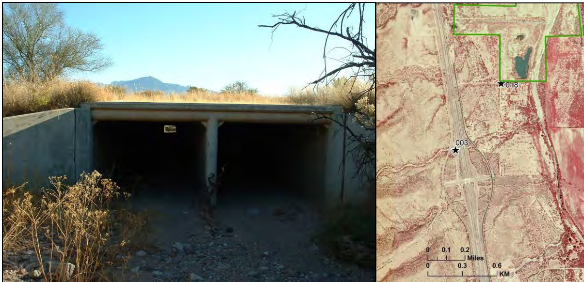
Figure 10: Looking east from waypoint 003 towards the Santa Rita Mountains, a 6 x 8 ft box culvert under I-19 and Frontage Rd. Waypoint 18 is at the southern edge of a Tucson Audubon Society conservation easement; a small rural housing area is south of waypoint 018. See Figure 5 to locate this scene within the linkage design.
