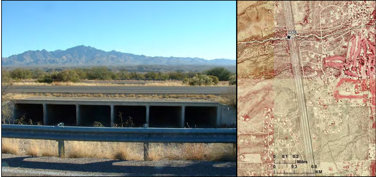
Figure 11: Looking east from Waypoint 004 towards the Santa Rita Mountains, Puerto Canyon crosses under I-19 via a set of six 7x9 ft box culverts. See Figure 5 to locate this scene within the linkage design.
