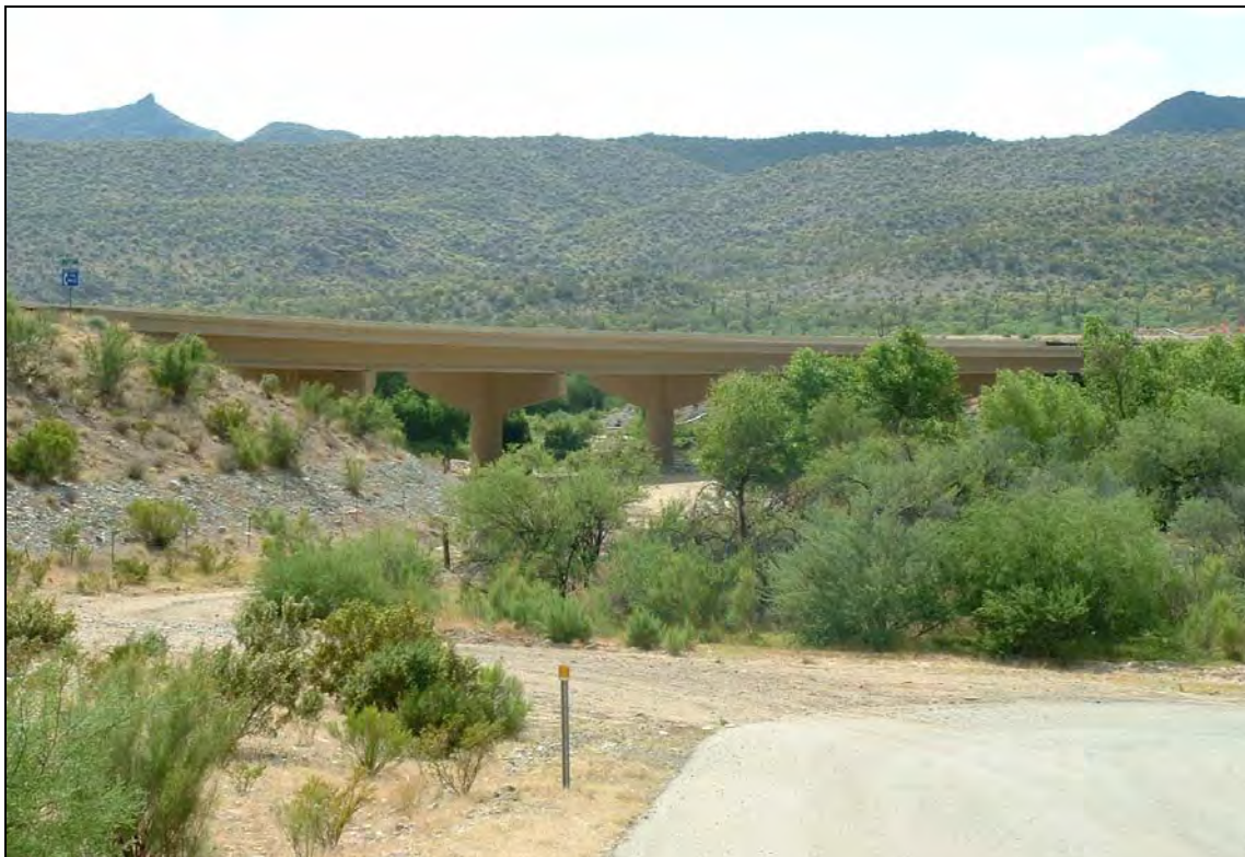
Figure 14: Looking north from waypoint 022, a large bridge 616' in width crosses over the Santa Maria River.
