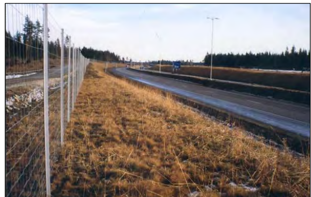
Figure 10: Potential road mitigations (from top to bottom) include: highway overpasses, bridges, culverts, and drainage pipes. Fencing (lower right) should be used to guide animals into crossing structures.
