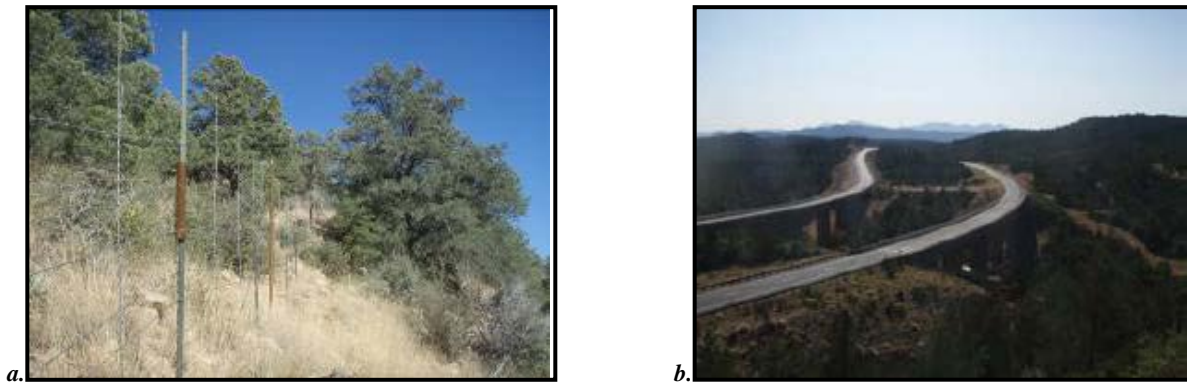
Figures 2a and 2b: Along Arizona State Route 260 near Payson, ungulate-proof fencing linking a series of highway underpasses effectively increased the permeability of the highway by 60% while reducing elk-vehicle collisions by greater than 80% at an estimated cost savings of $1 million dollars annually (Dodd et al. 2007; Photographs: Arizona Game and Fish Department).
